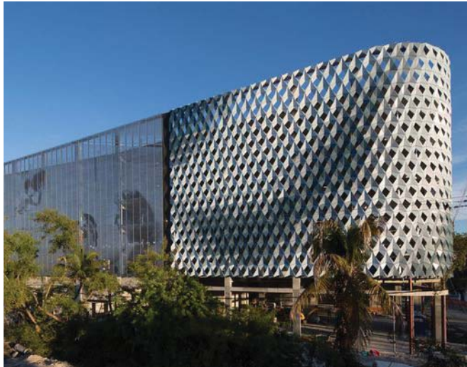
eastland shopping centre louvred carpark facade provides natural ventilation
