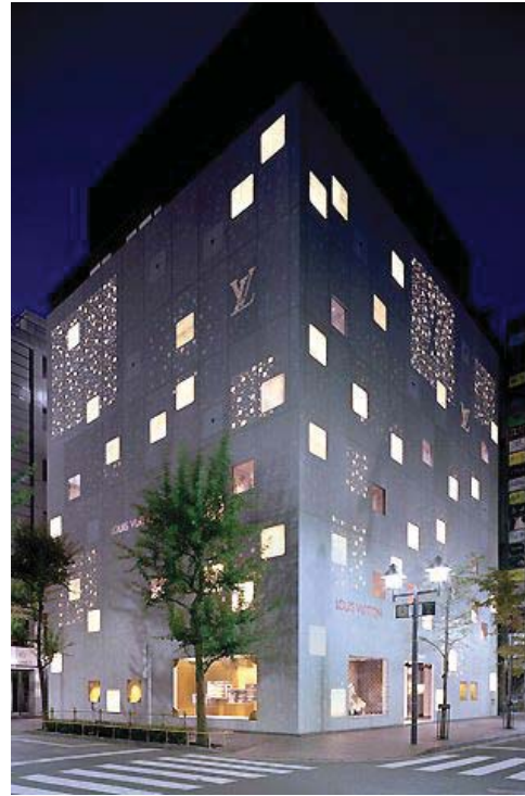
design penetrations in precast concrete so the building can take on another form at night
