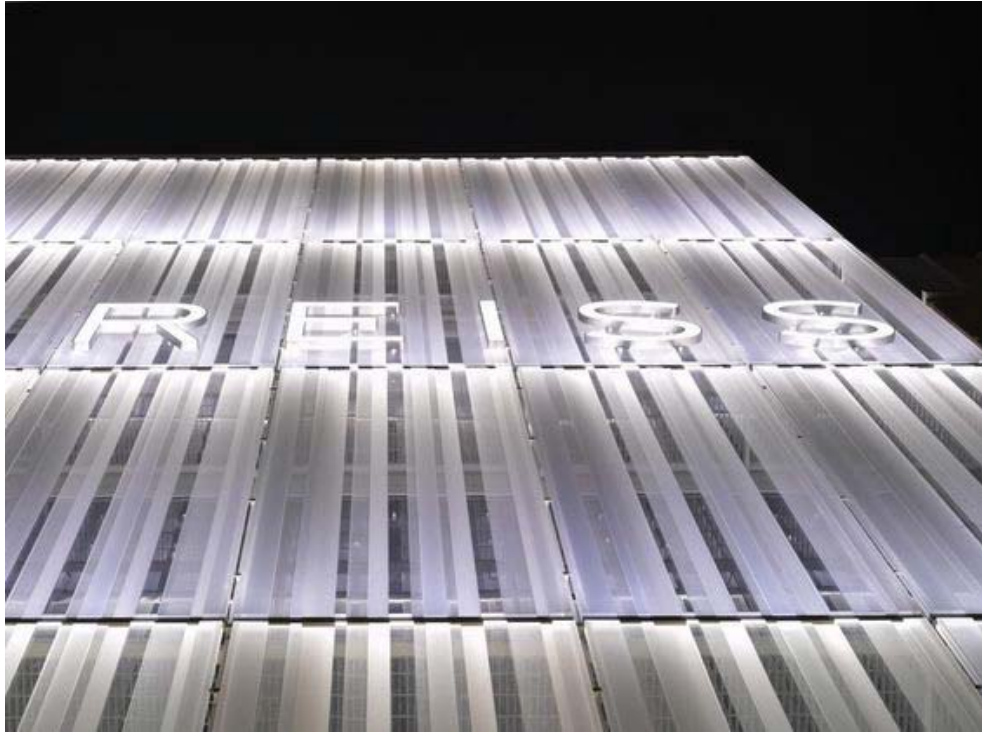
layering facade provides a sense of permeability
