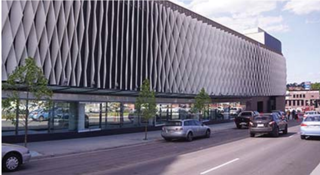
eastland shopping centre louvred carpark facade provides natural ventilation
